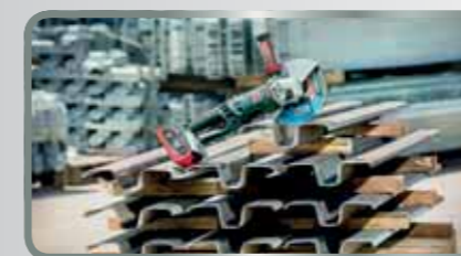
Cutting through 11 crash barriers Material: Sheet steel
