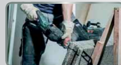
Sabre saws can, thanks to the universal range of sabre saw blades, be used in different materials, such as here in aerated concrete.
